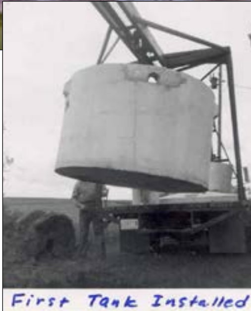
1965 First Tank Installed: Joe Wieser installed the first tank in 1965 for Clem and Isabel Horn in rural Maiden Rock.
