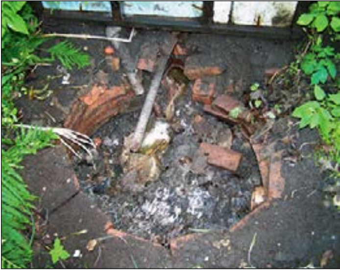
Organized residents and funding are vital components to bringing noncompliant rural sewer systems into compliance.
